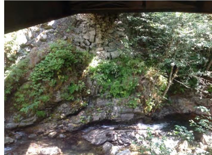
Left Bank Abutment when facing downstream
