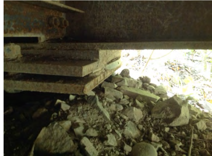
bearing plates and pads - typical
