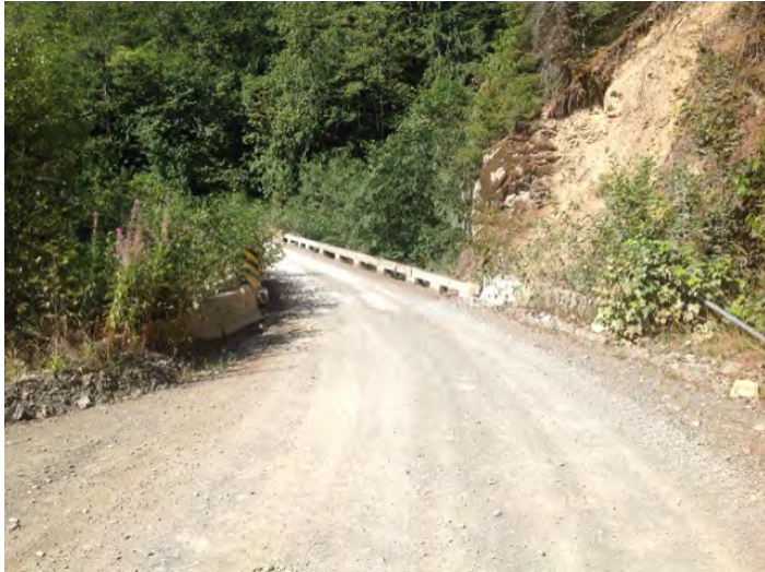
Approach from Left Bank when facing downstream
