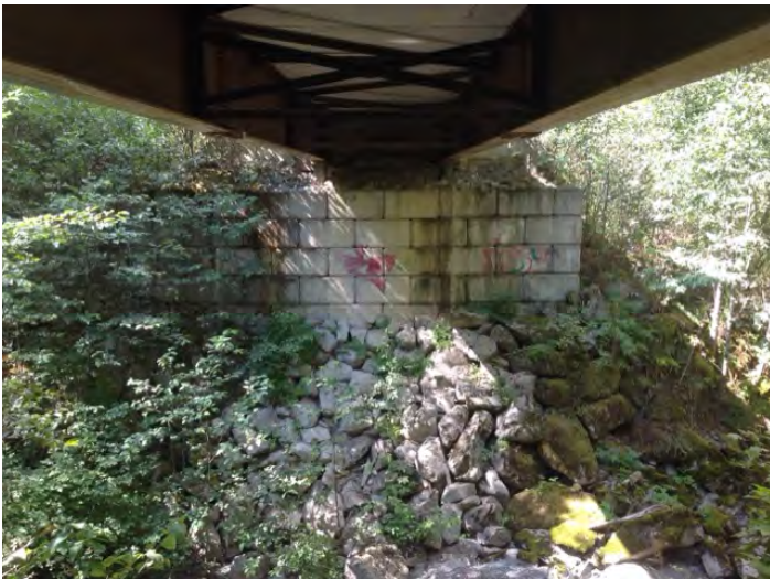
Right Bank Abutment when facing downstream
